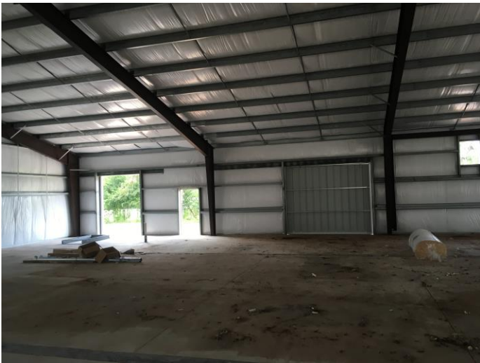
3. Sliding door installation at Small Animal area
