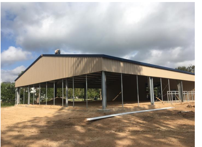
6. PEMB at north elevation
