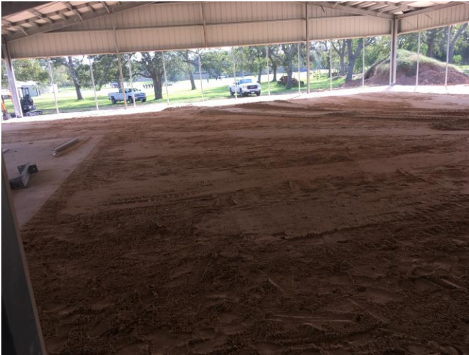
1. Installation of livestock soil at Large Animal area
