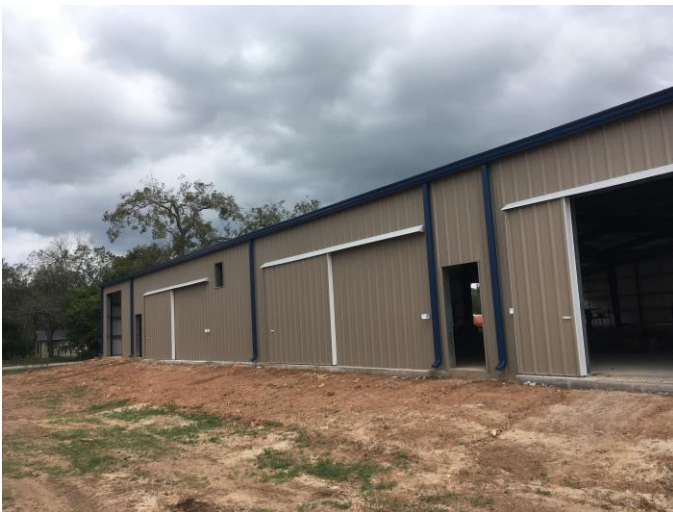
5. Sliding doors at west elevation
